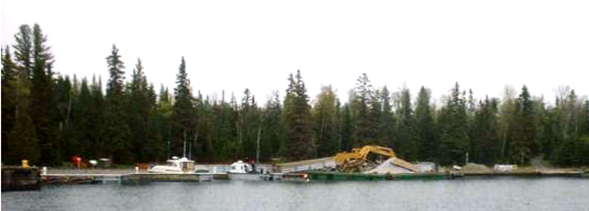
Dock repair at Rock Harbor, 2001
